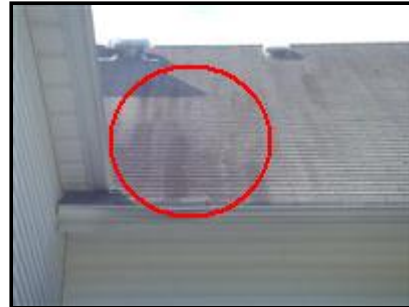
1.0 Picture 2 Rear roof stains,which can be professionally removed
